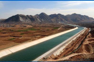
The 3 - 1000 km long water S/N transfers diverting flows of the Yangtze river to provide water to the water stressed cities of Beijing and Tianjin in the Hai river basin.
