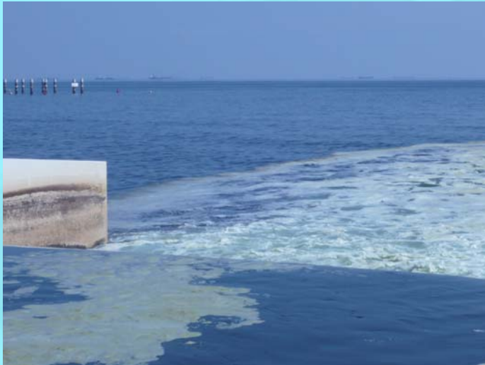
Outfall of Fujairah power plant.
