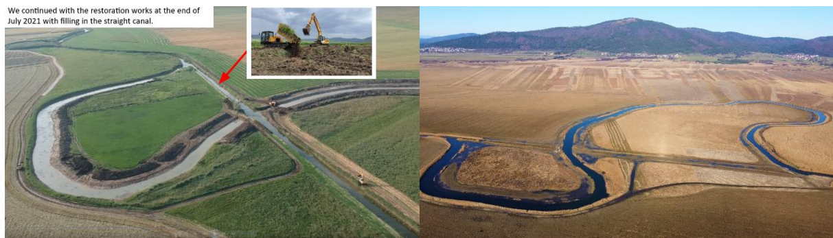
Figure 3: restoration works at the end of July 2021 with filling in the straight canal (left)/after restoration works (right)
