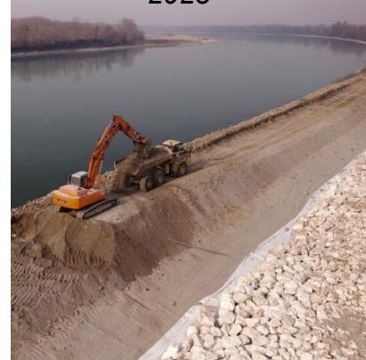
Lowering river groynes to restore lateral connectivity
