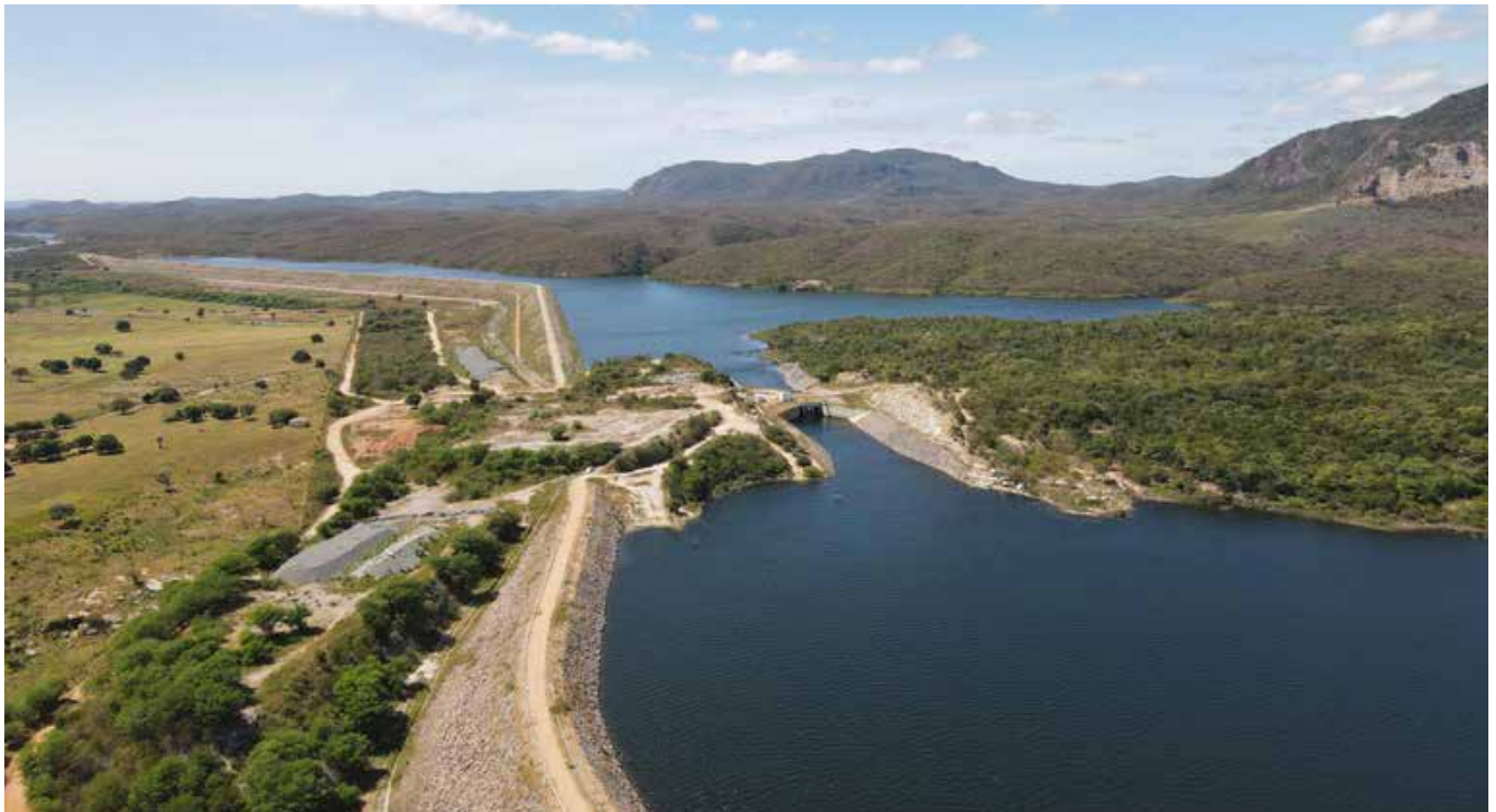
São Francisco River Integration Project (PISF) © MIDR
