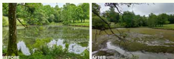
Work to remove ponds in the Vienne Basin with the aim of restoring hydrological continuity © EPTB Vienne
