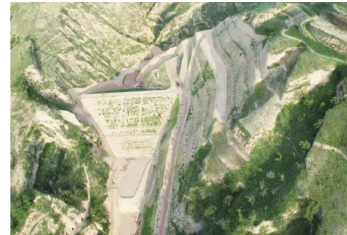
Rigid check dam
