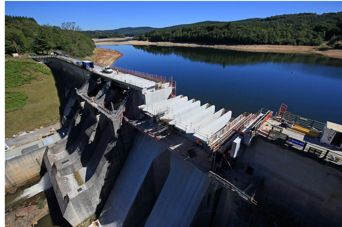
The Raviège Dam, in the Tarn
